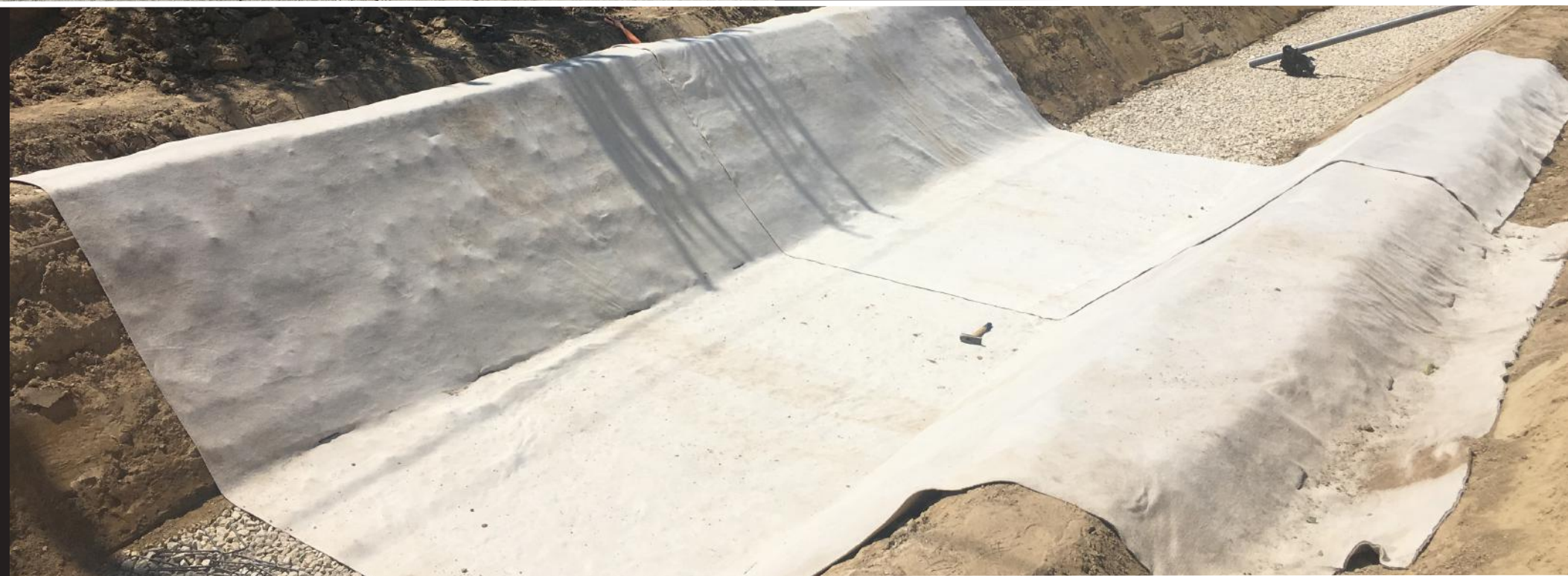
CANAL AND DITCH LINING
