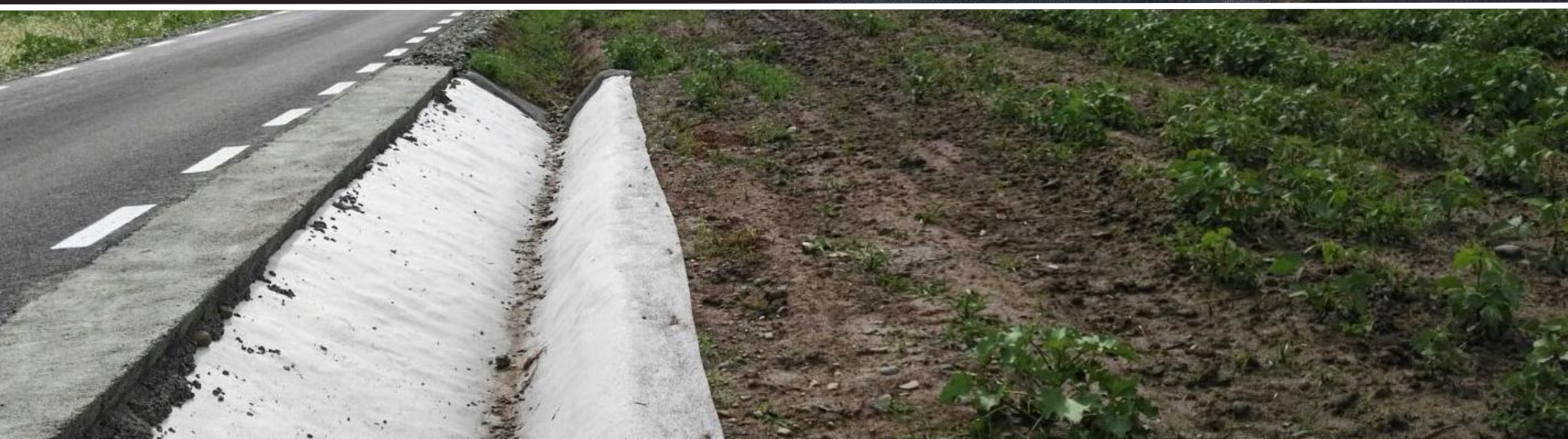
ROAD AND RAILWAY DITCHES LINING
